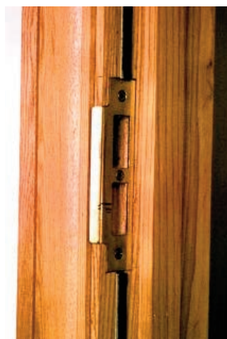
Smoke seals interrupted by lock strike
